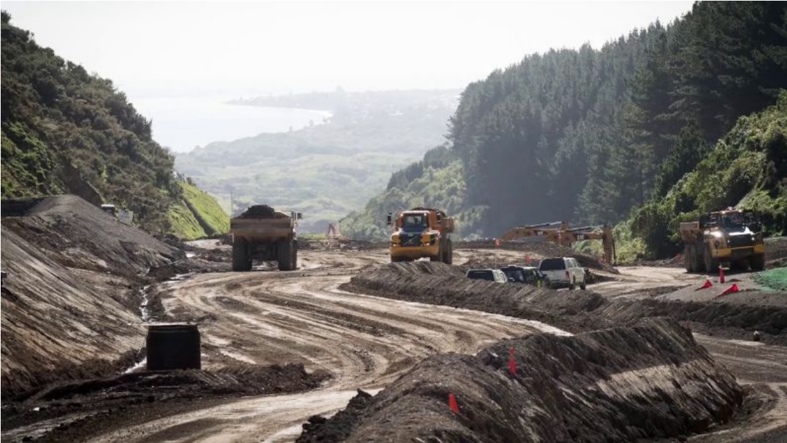
Transmission Gully - Photo courtesy of NZTA.
